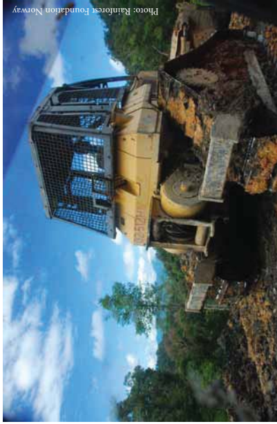
Bulldozer at work, Malaysia.
